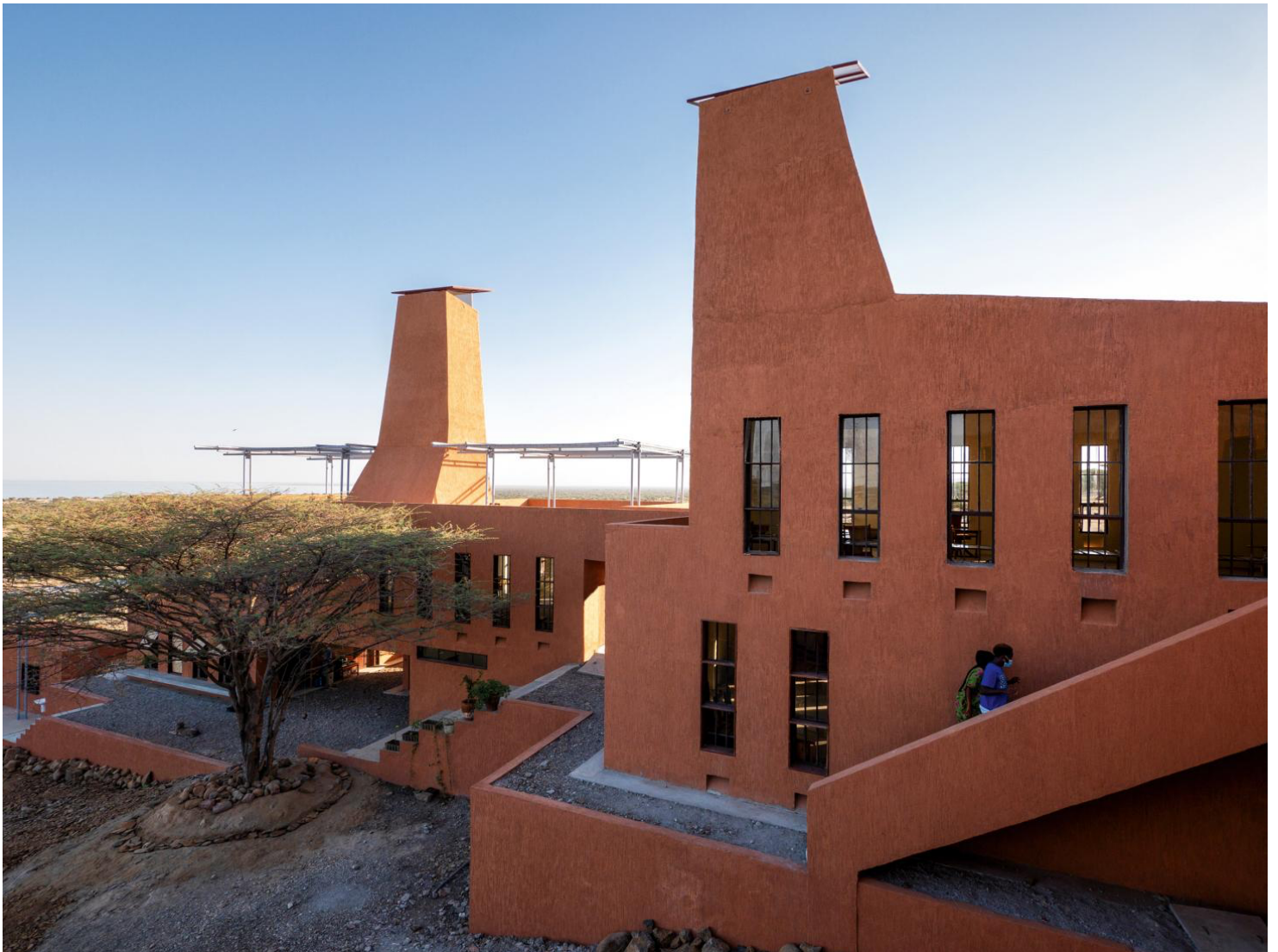
The Slak education campus in Kenya's Turkana County, by Kéré Architecture, is Aitken's pick for Best Public Building in
